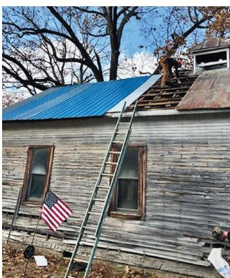
*In one of the first steps of the restoration, Dustin Eveland and Keith Strickland remove and replace the metal roof.*
